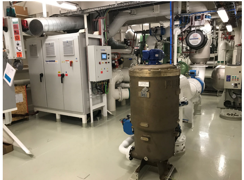
The HG1000U system can be supplied as loose components, enabling more flexibility in terms of installation space and configuration.
