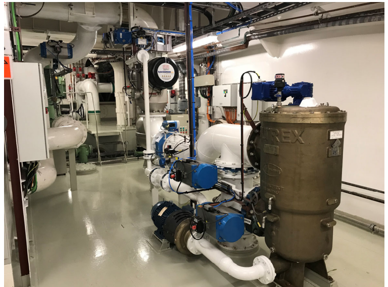
The HG750U system can be supplied as loose components, enabling more flexibility in terms of installation space and configuration.
